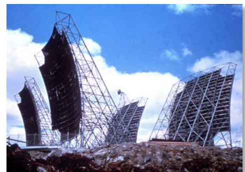
Above: Northern CNCP microwave repeater station. CRC Image 79-38692
