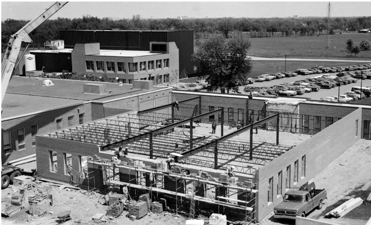
Construction of Bldg. 34 at Shirleys Bay in 1974, CRC Image 74-29767
